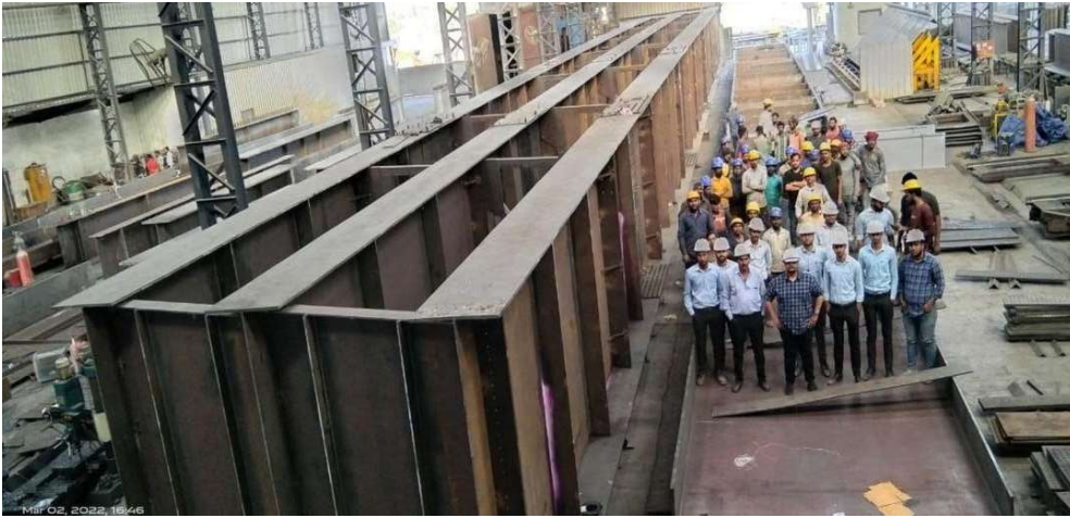
ASSEMBLY OF 57.5 MTR OF STEEL PLATE GIRDER & LAUNCHING. CR, NAGPUR DIVISION
