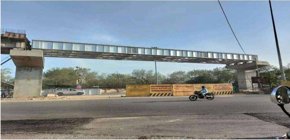
35 MTR. SPAN AT JHOTWARA FLYOVER PROJECT, JAIPUR, JAIPUR DEVELOPMENT AUTHORITY
