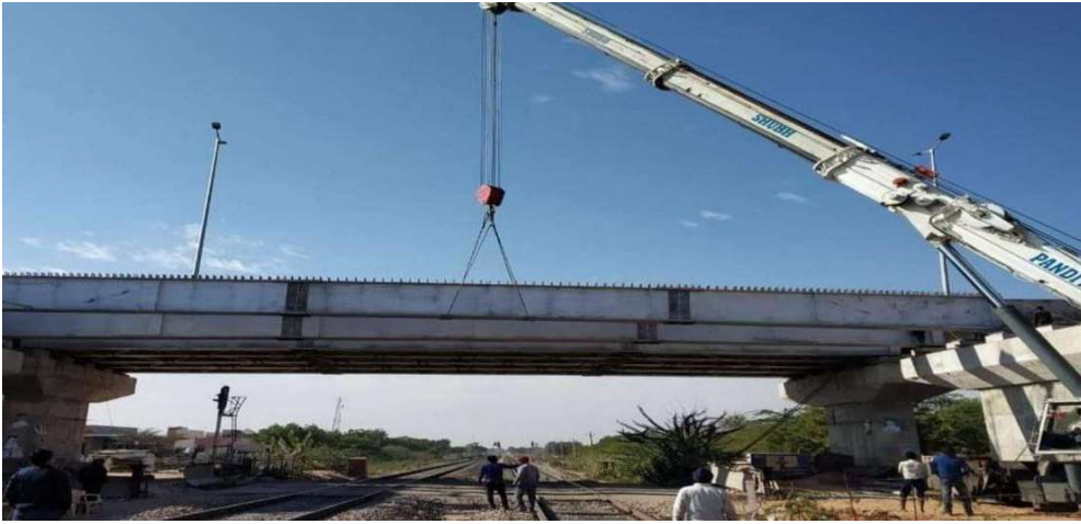
30 MTR. SPAN IN LIEU OF LC-57, PHALODI, IRCON, NWR JODHPUR DIVISION
