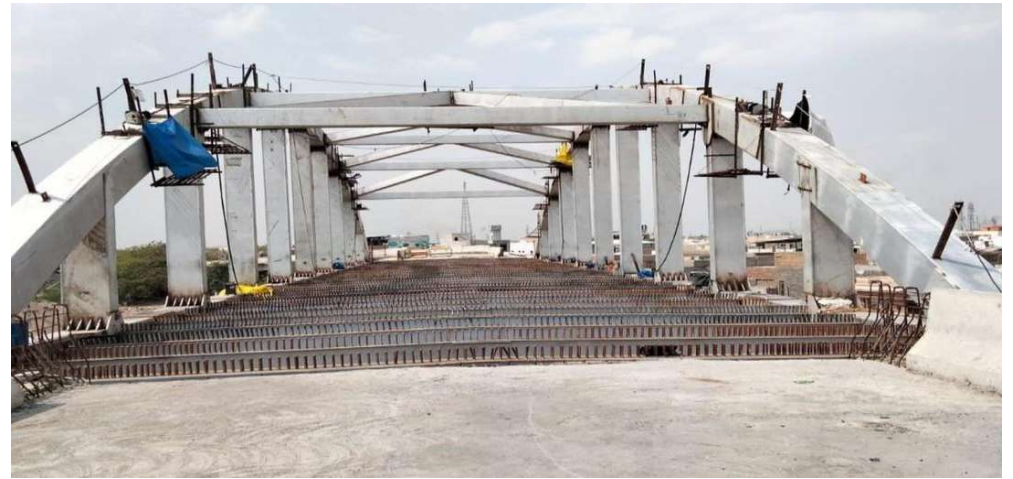
62 MTR. BOW STRING GIRDER LAUNCHING
