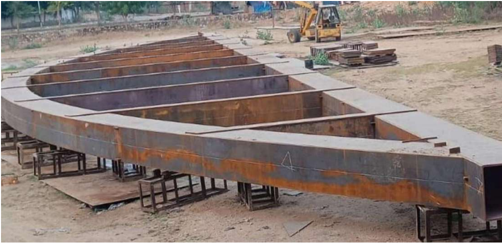
62 MTR. BOW STRING GIRDER ASSEMBLY AT FACTORY
