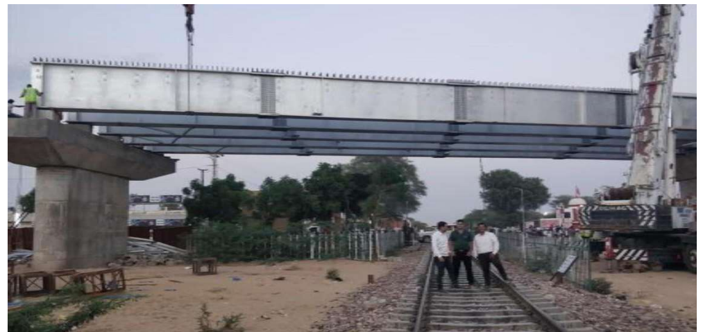
36 MTR. SPAN IN LIEU OF LC- 06, NAL, BIKANER, IRCON, NWR BIKANER DIVISION
