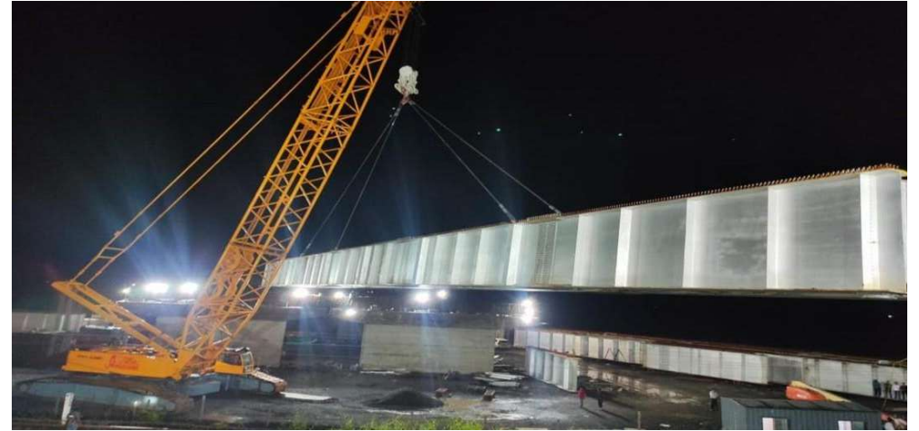
ASSEMBLY OF 57.5 MTR OF STEEL PLATE GIRDER & LAUNCHING. CR, NAGPUR DIVISION
