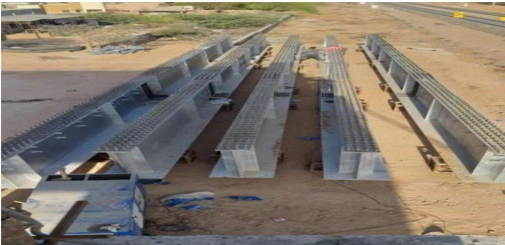
36 MTR. SPAN IN LIEU OF LC- 06, NAL, BIKANER, IRCON, NWR BIKANER DIVISION
