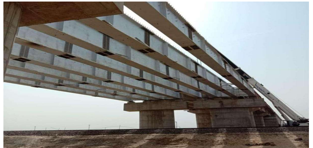
36 MTR SPAN ROB DIDWANA RAJASTHAN, NWR, JODHPUR DIVISION
